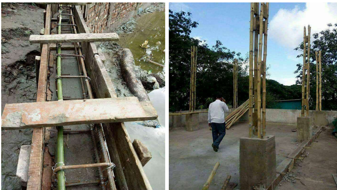
Figure 2: Bamboo used to reinforce concrete in beam and columns
