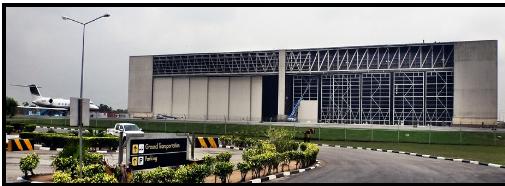
Figure 3 Maintenance Repair and Overhaul Hangar - Uyo Airport
