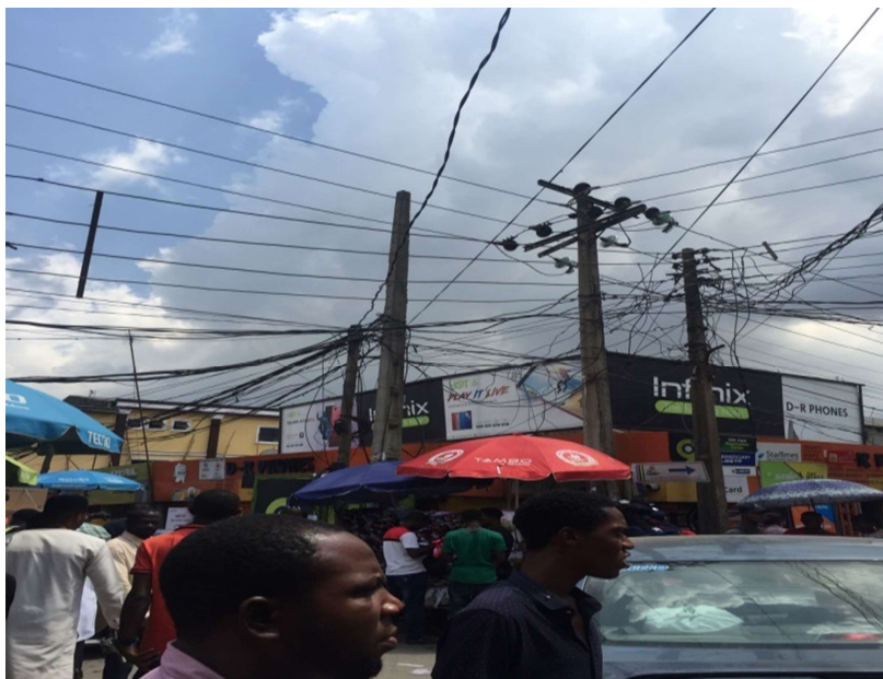
Plate 4: Haphazard electric cable connection
