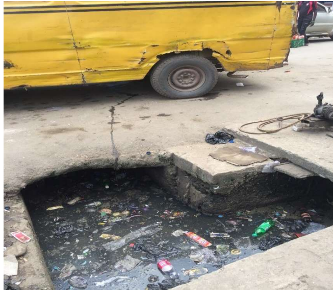
Plate 2: Poor condition of the drainage
